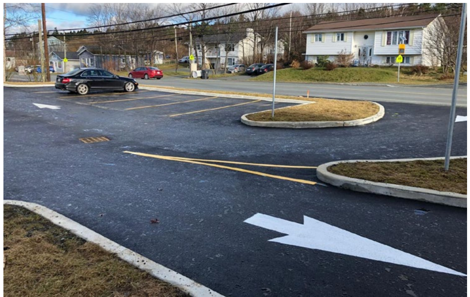
Parking Lot @ 2750 Topsail Rd. (Nov. 2020)
